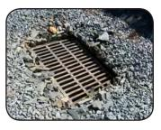
Figure 55. Drainage tiles lead to underground pipes that carry water to the containment structure
